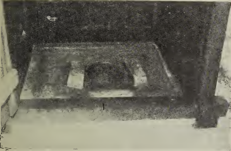
II. Concrete Squatting Platform to No. I.
