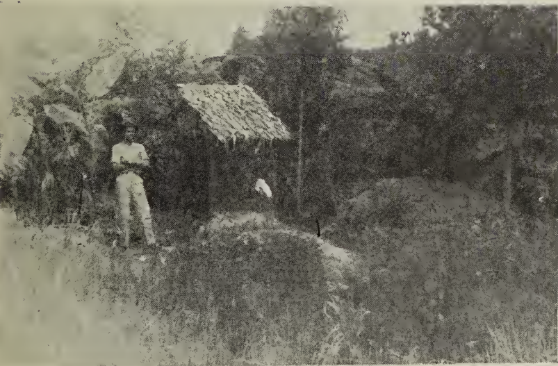
III. Original-Latrine of the same construction but of a cheaper type compared to No. 1. Note the handkerchief—the position of the pit.
