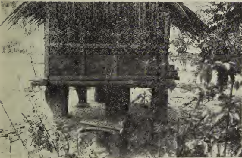
IV. Similar type of Latrine, having the flushing tube above ground (X) the position of the pit.
