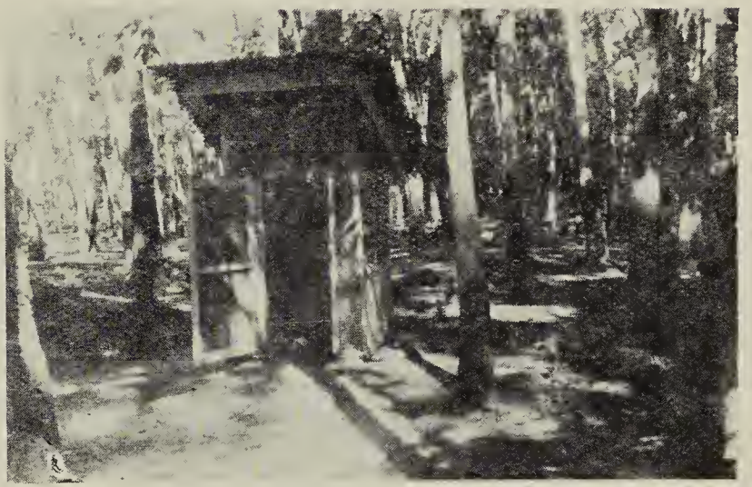
Pit Latrine with concrete squatting platform.
